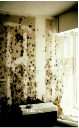
Invisible mold due to high humidity within the building envelope
