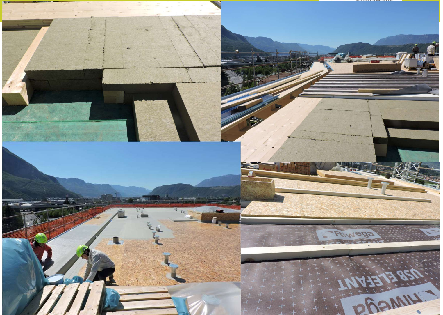
Roof insulation
