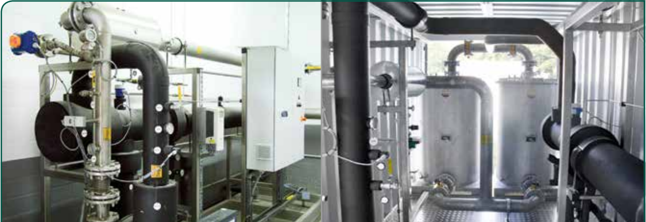
PlanET gas drying and cleaning system | Container solution with activated carbon filter
