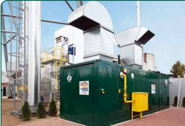
Containerised CHP | CHP in engine room
