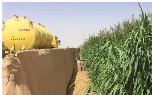
Nature-Based Solutions: A yellow tanker discharging raw sewage and sludge into a constructed wetland designed and constructed by BAUER Resources GmbH.
