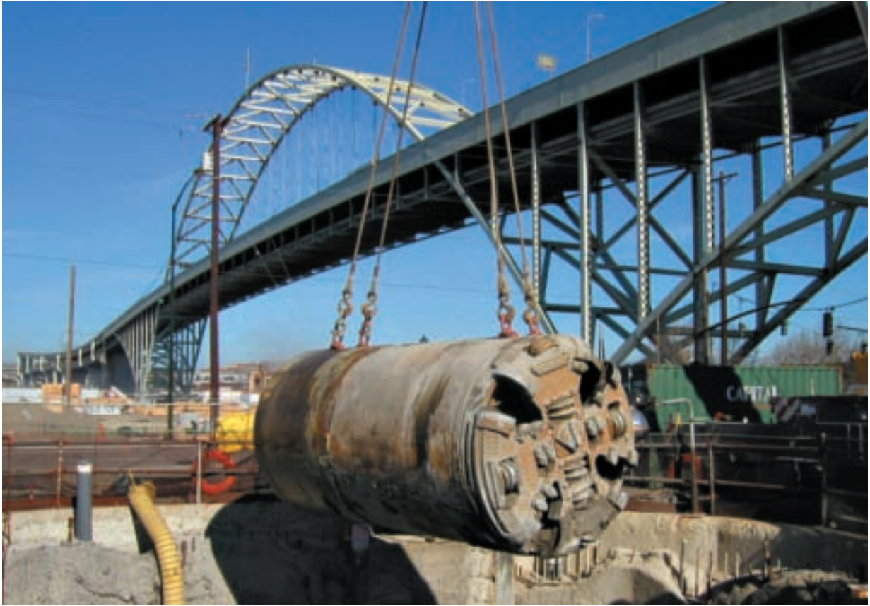
Small diameter tunnel boring machines are realizing new sewage tunnels, for example for the CSO in Portland.
