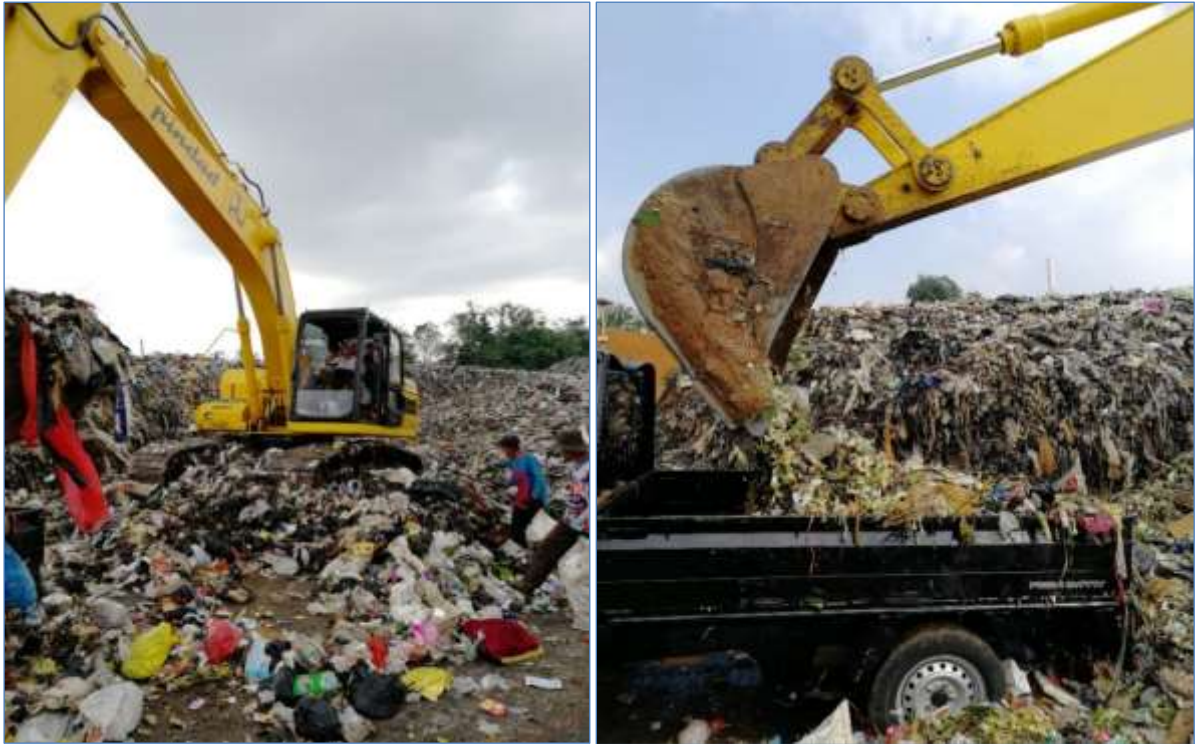
Figure 6: Mixing and moving waste from area A to area B
