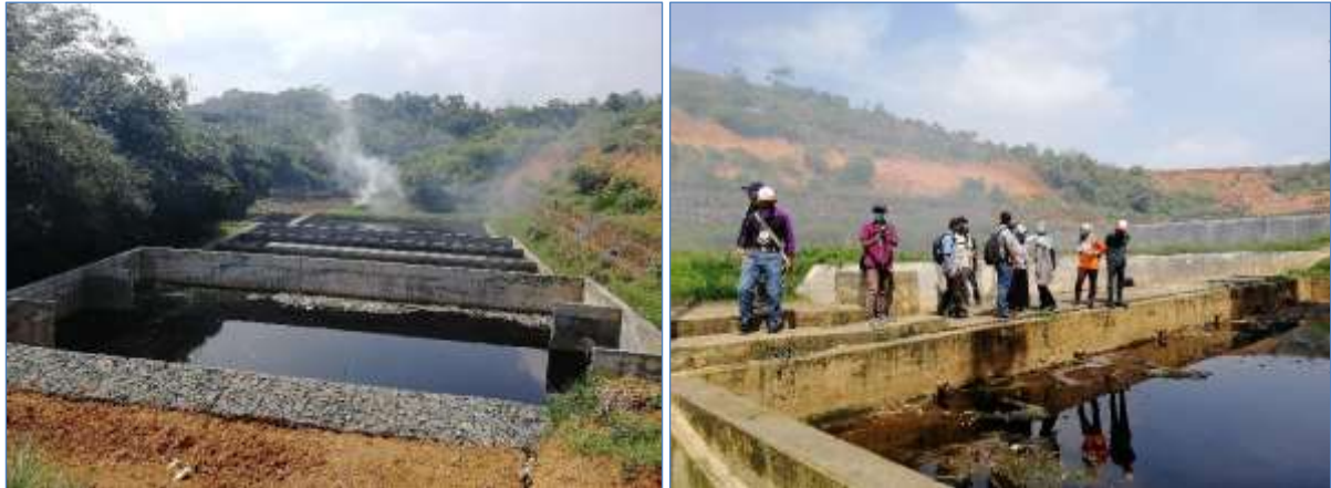
Figure 7: Leachate water treatment system in Ciangir landfill site
