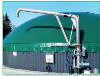
By installing individual components, it is also possible to equip the **barrel filling station** with several options. It can be set up as being height adjustable, can be equipped with a hand pump and, if requested, with a remote control.
