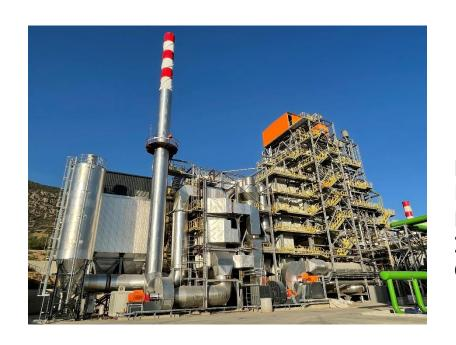
**Firing Capacity**: 40 MW Electrical output: 13.5 MWel, **Fuel**: Textile, chicken litter
