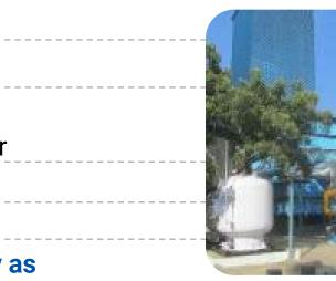
HYDERABAD, INDIA 2022-present  $0.4 \text{ MW}_{\text{th}}$ 600 m<sup>3</sup> syngas/hour Pharmaceutical waste 0.15 ton/hour Fuel used industrially as natural gas replacement
