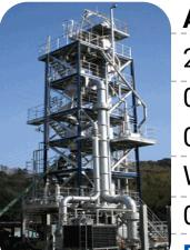
ANAN, JAPAN 2006-2009  $0.15 \text{ MW}_{\text{th}}$ 0.038 Mw<sub>e</sub> Woodchips 0.1 ton/hour **Demonstration plant**
