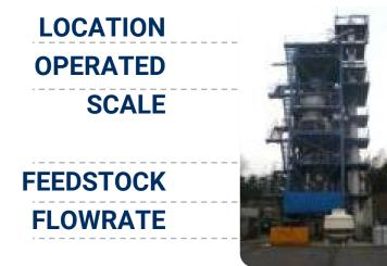
IZUMO, JAPAN 2005-present 1 MW<sub>th</sub> 8.92 kg H2/hour Woodchips 0.6 ton/hour **First commercial plant**
