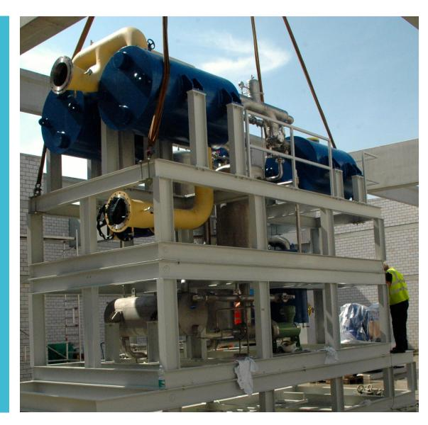
Cooling capacity: 950 kW **Ammonia condensation** with booster:  $+55/-7^{\circ}$ C Hot water in/out: 95/80°C Cooling water in/out: 26/31°C COP = 0.4 App: frozen food store **Ammonia direct condensation via ammonia tank**
