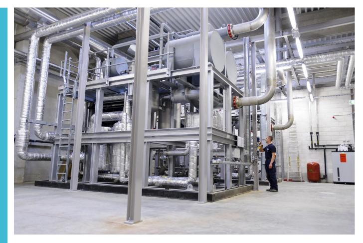
Cooling capacity: 800 kW **Ammonia condensation** with booster:  $+55/-7^{\circ}C$ Hot water in/out:  $95/80^{\circ}C$ Cooling water in/out:  $26/31^{\circ}C$ COP = 0.4 App: frozen food store
