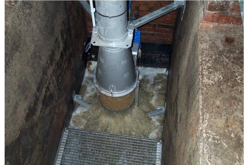
HUBER ROTAMAT® RoK4 for small Pumping Stations
