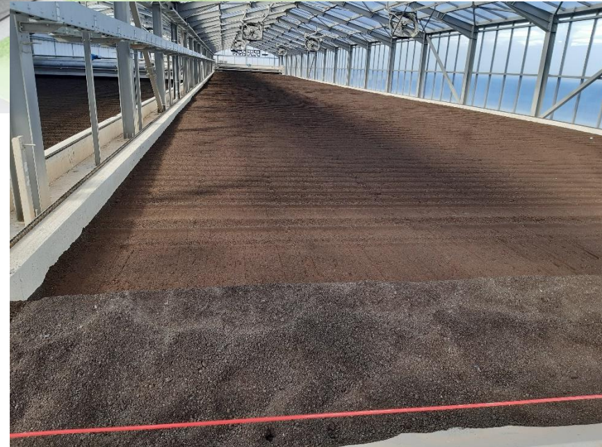
Solar Sludge Dryer WWTP Rethymno
