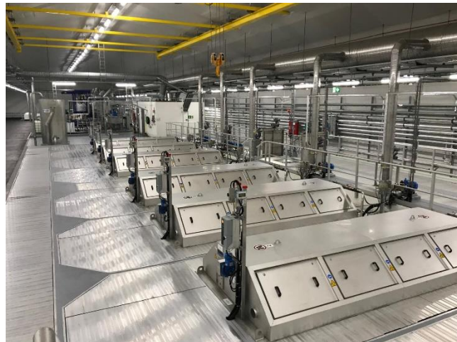
HUBER Drum Screen LIQUID® Primary Clarifier Replacement and Membrane Screening
