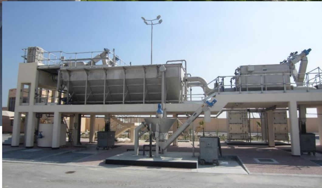
Ro5 Package Headworks followed by a membran screen
