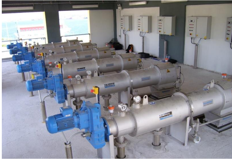
sludge screen with SP4 WWTP Psytalia
