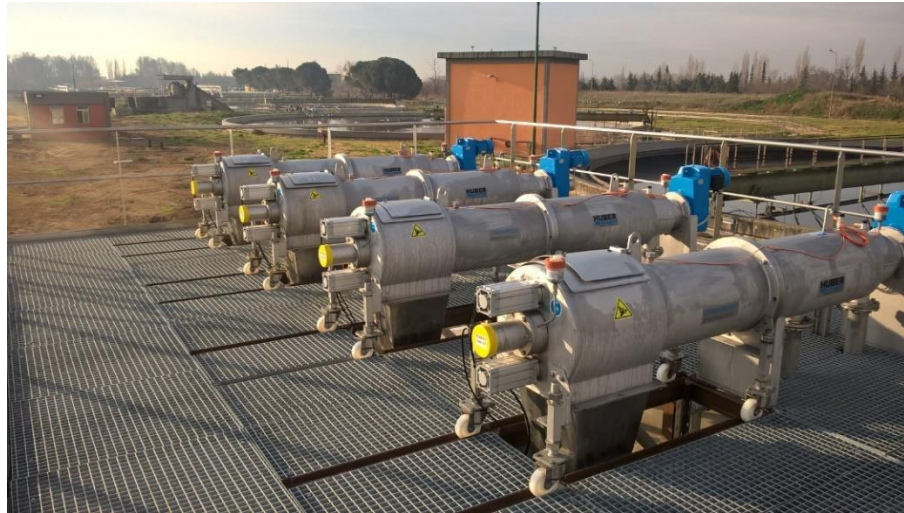
Sludge Screening with the HUBER Strainpress® WWTP Sindos
