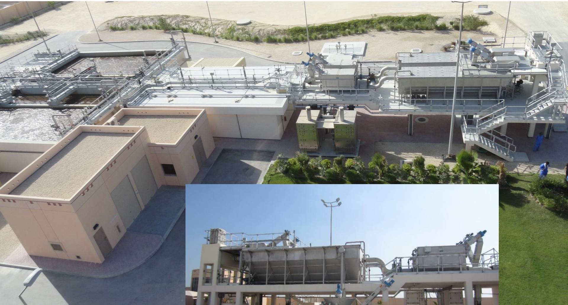
Ro5 Package Headworks followed by a membran screen
