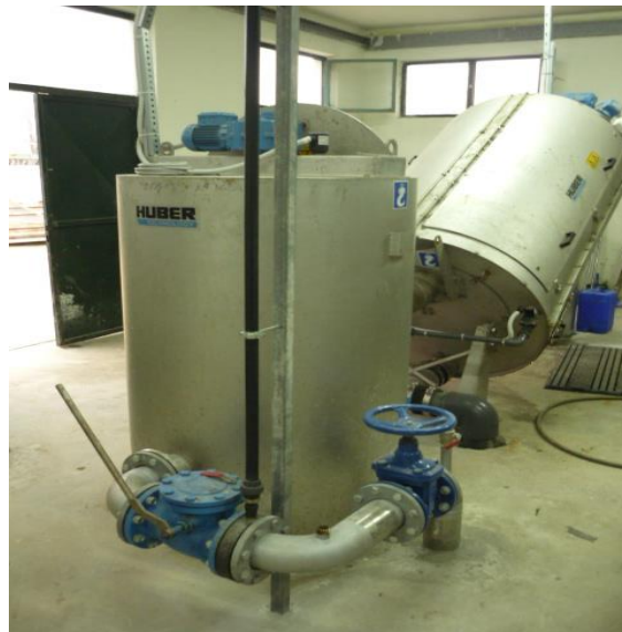
Sludge Thickening with HUBER S-Drum® Thickener WWTP Volos
