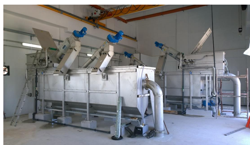
HUBER Complete Plant ROTAMAT® Ro 5 WWTP Aegion
